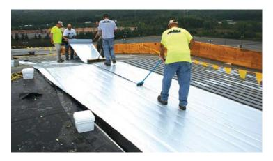
**Use the proper Versico-approved details.** It is not uncommon to see non-traditional details used on AVB installations. It is critical that AVBs are properly sealed per Versico specifications and details.
